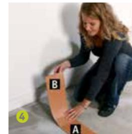
Continue to install the remaining floor to ends of the room, taking care when cutting planks or tiles to fit along all walls.
