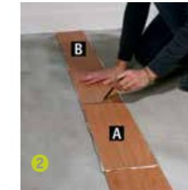
Install the first plank or tile from this central point towards the adjacent sides of the room.
