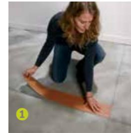
Identify and mark the centre point of the room by drawing two perpendicular lines on the floor.
