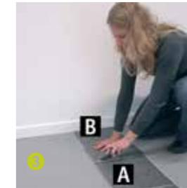
At wall, draw and then cut the tile to the correct size.
