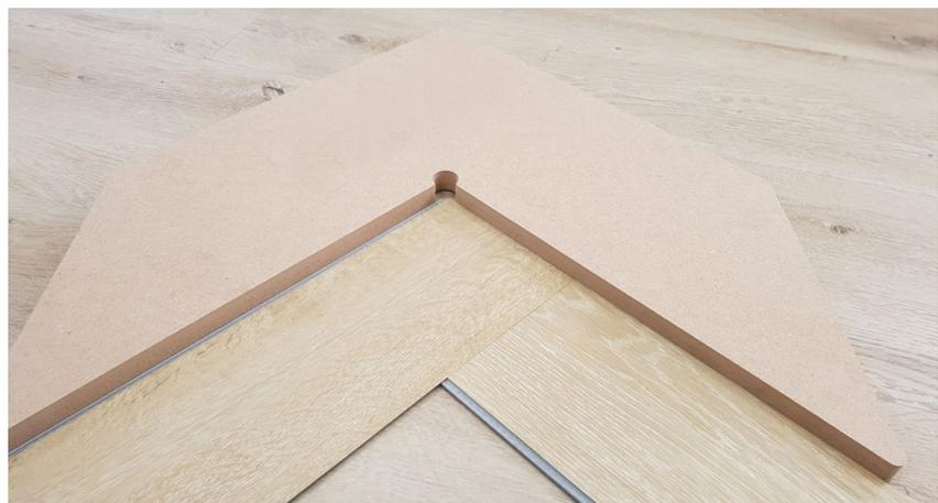
Simplify the cutting and fitting of herringbones planks with the use of a T-square.
